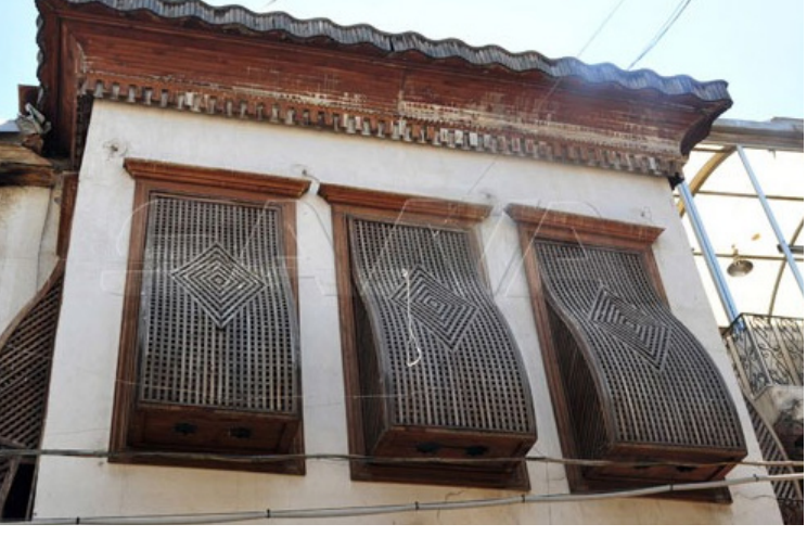
Mashrabiya Latticework for privacy, shading and ventilation
